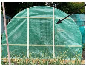
On the outside two more pieces of wood were fixed and screwed though to the inside, sandwiching the cover between them. For extra security batons were fixed to long edge sides from the inside using more pipe clips. Around the bottom the cover was dug into the ground and sandwiched between wood screwed to the base frame.
