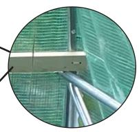
Two holes drilled and a cable tie fitted through and round the frame.
